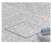
Laying the floor covering in the RKN cassette Lay the floor covering in the cassette and stick it down. Seal the remaining gap between the floor covering and the cassette with suitable materials.
