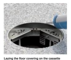
Work the floor covering to the cassette frame. Seal the remaining gap between the floor covering and the cassette frame with suitable materials.
