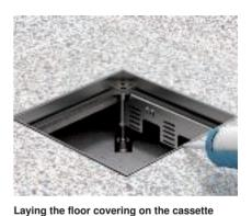
Work the floor covering to the cassette frame. Seal the remaining gap between the floor covering and the cassette frame with suitable ma-
