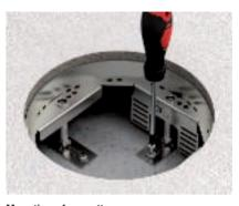
Mounting of cassette Fasten the levelling units of the cassette on the raw ceiling.
