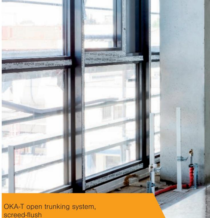
The open, screed-flush OKA-T trunking system is used for cable routing and the installation of electrical resources in the underfloor area. The trunking system is closed on all sides. It can be opened along the entire length.
