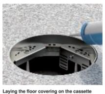
frames Work the floor covering to the cassette frame. Seal the remaining gap between the floor covering and the cassette frame with suitable ma-
